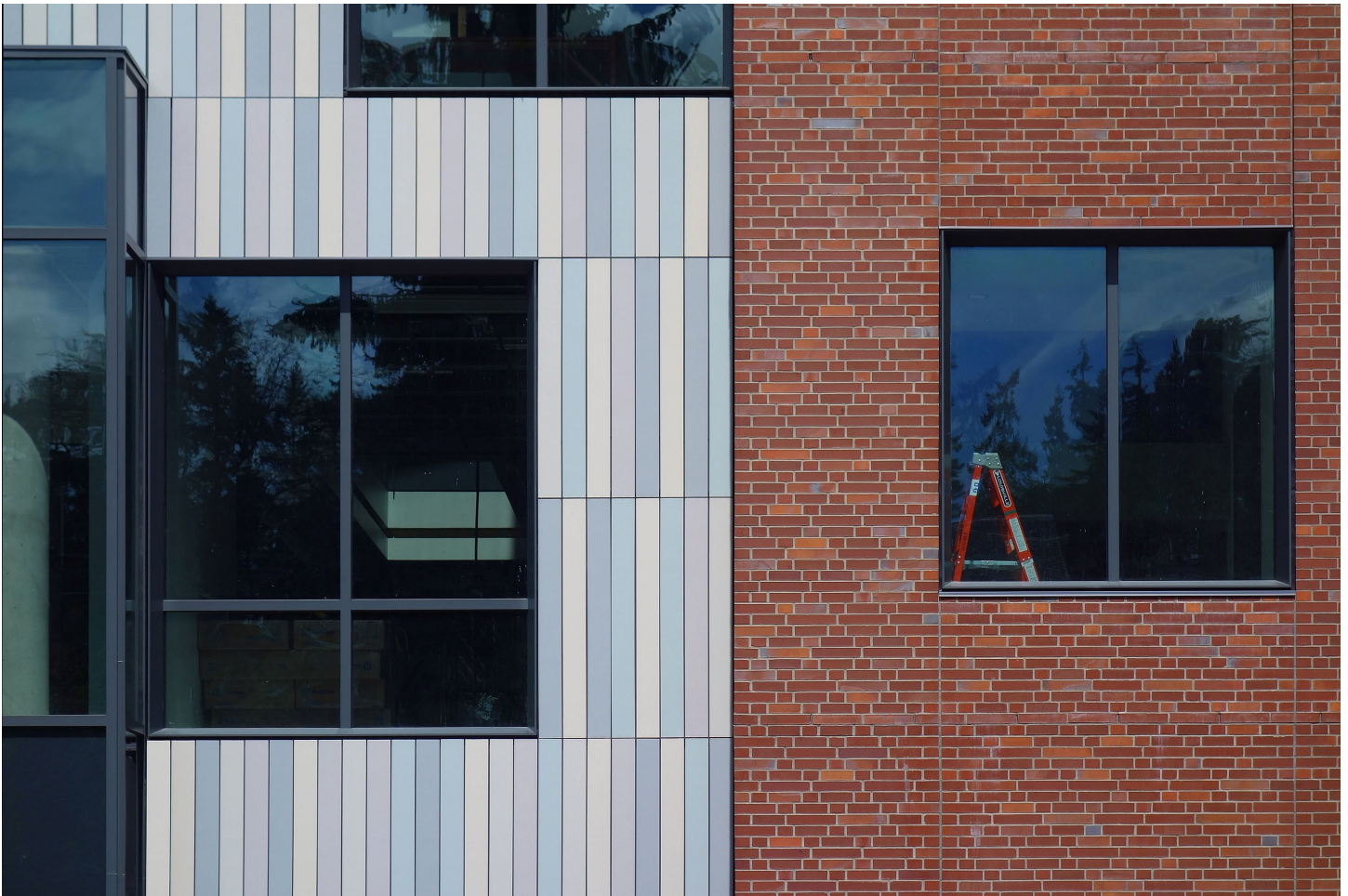
Construction Image of UO Tykeson Hall, detail of terra cotta, custom brick pattern, and curtain wall glass, Photo M. LaFoe, 2019.
