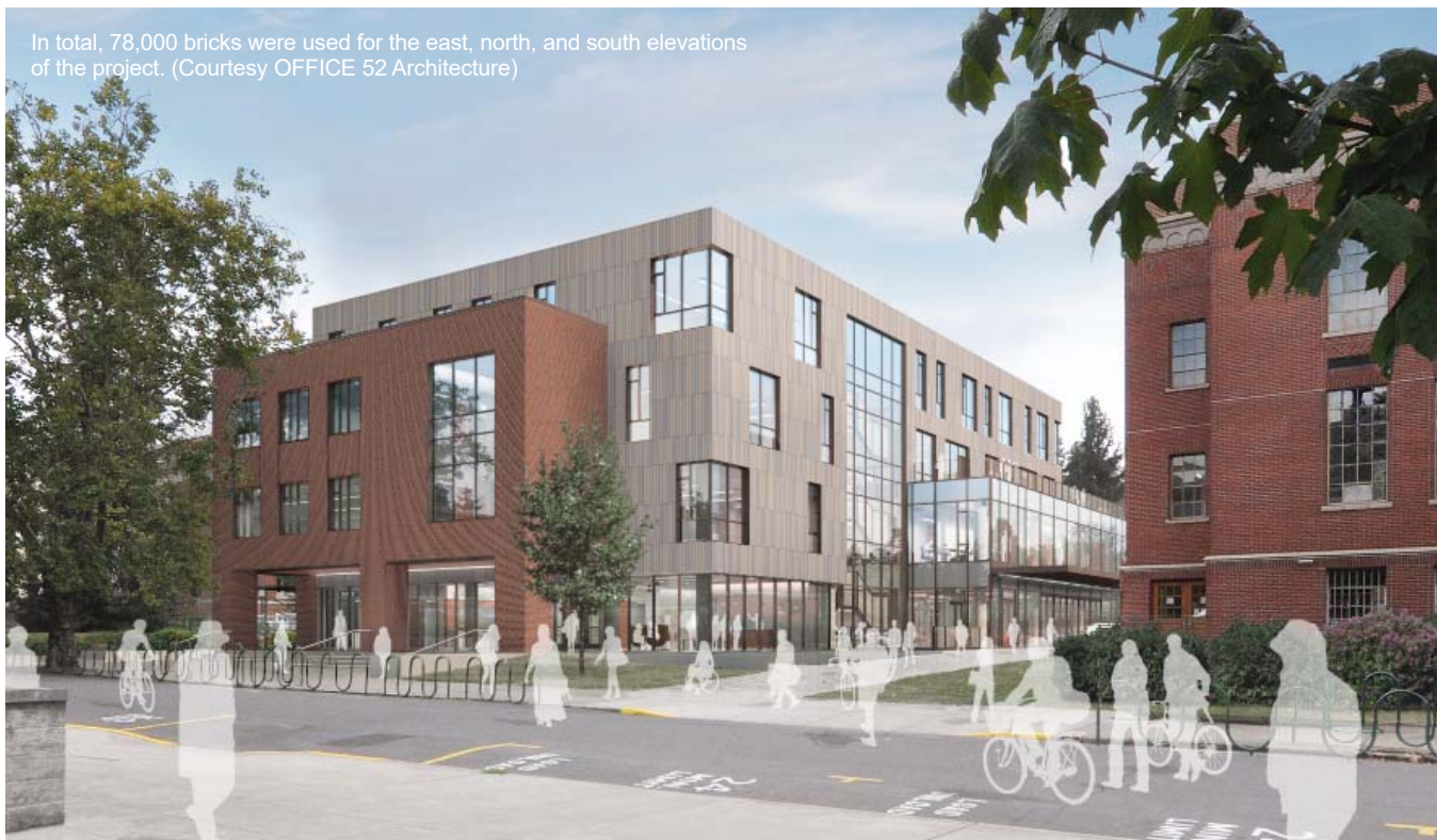
There are significant stretches of glass curtainwall found along the facade. (Courtesy OFFICE 52 Architecture)
