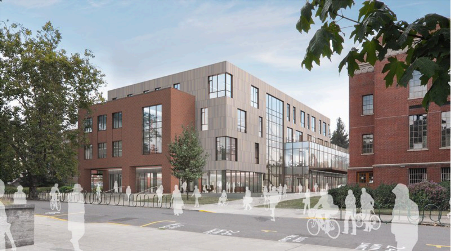
Construction is currently underway for the Willie and Don Tykeson Hall at the University of Oregon (UO) in Eugene. Photo Credit: OFFICE 52 Architecture
