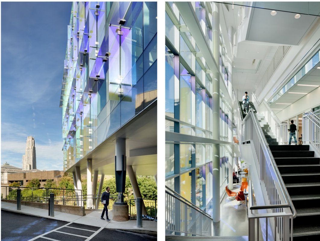
Detail, South Façade (left), Interior Collaboratory public space (right), Carnegie Mellon University Scott Hall, Photos by Jeremy Bittermann, Courtesy OFFICE 52 Architecture.
